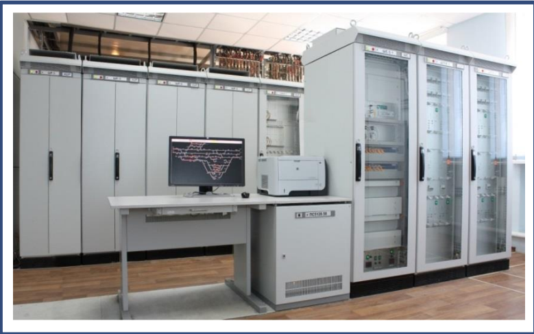
MPC-U equipment in the «relay» room of the electrical interlocking post
